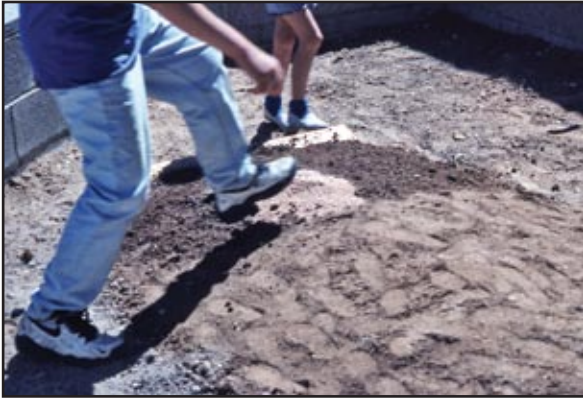
Figure 17. Mounded, packed rock-free soil helps keep out the rain.
